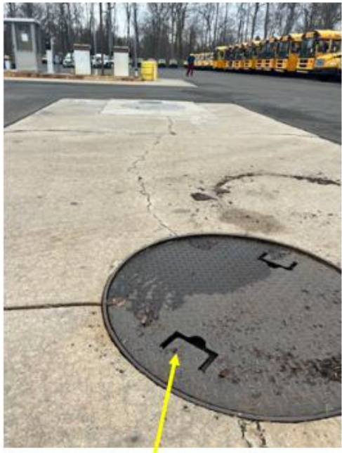
(1) Manhole removal and replacement.
